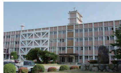
本館(1号館) Main Building
