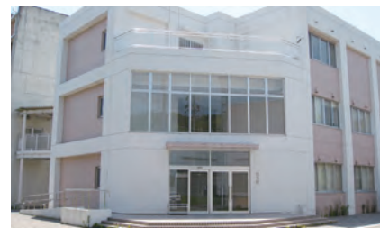
4号館 No.4 Building
