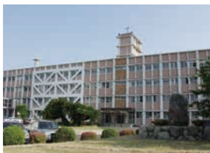
本館(1号館) Main Building
