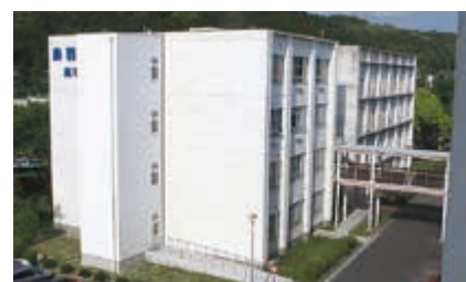
校舎(3号館) No.3 Building
