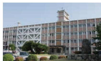
本館(1号館) Main Building
