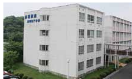
校舎(3号館) No.3 Building
