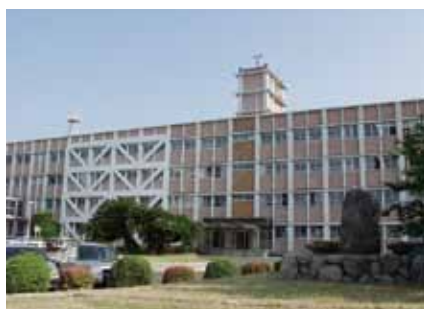
本館(1号館) Main Building
