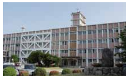
本館(1号館) Main Building
