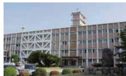
本館(1号館) Main Building
