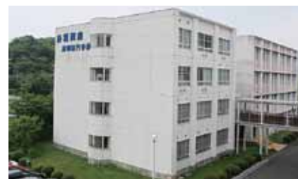
校舎(3号館) No.3 Building
