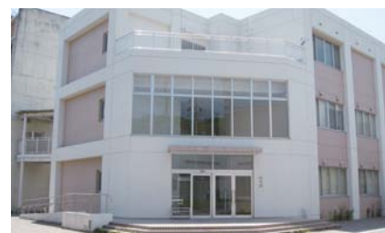
4号館 No.4 Building
