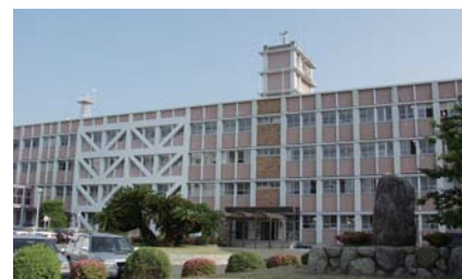
本館(1号館) Main Building
