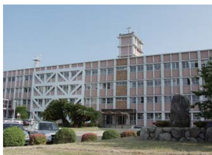
本館(1号館) Main Building
